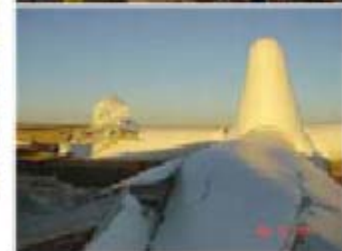
Japan - January 2007 69 metre wind turbine - In Service since 2001 Collapses in 28 km/h wind
